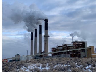
Power Plant for Electricity Generation
