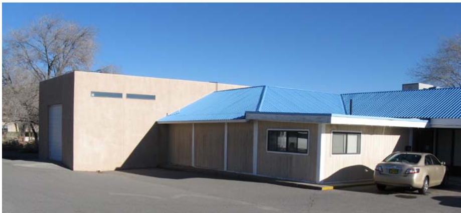
Outside View of Dr. Thomas Claytor's Lab in White Rock, NM
